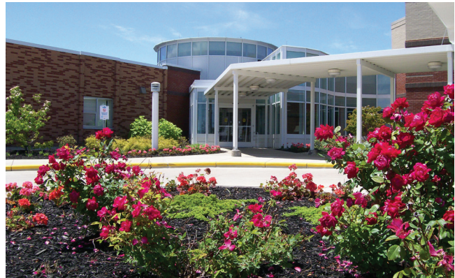
Rehabilitation Center Entry (Phase II)
